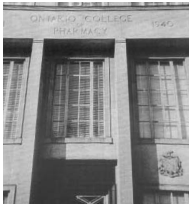
Former Ontario College of Pharmacy offices at 44 Gerrard Street East, Toronto
